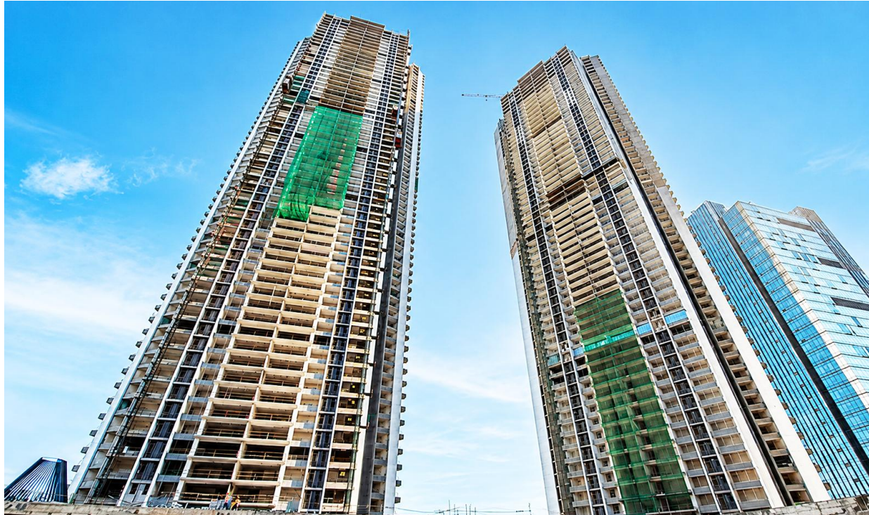
Towers – A & B
