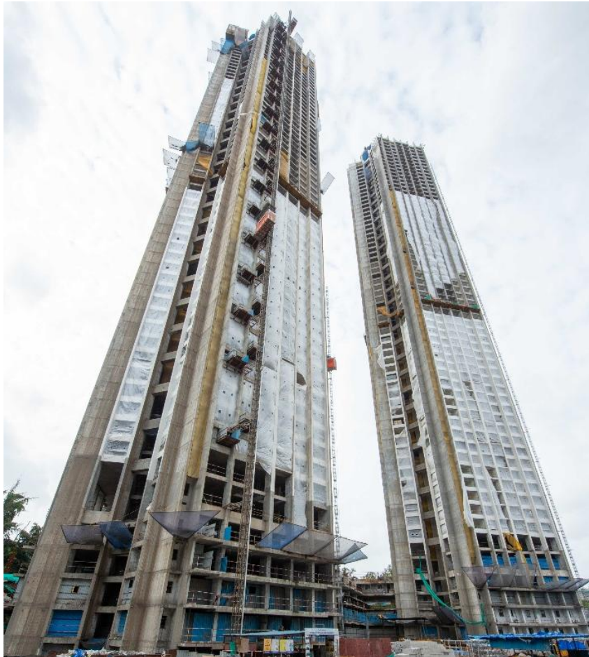
Towers – B & C
