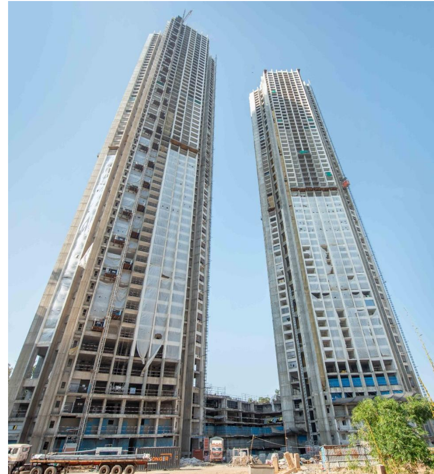
Towers – B & C
